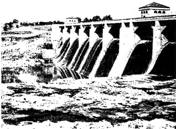
Fig. 8.—O'Shaughnessy Dam built in 1925 near Columbus, Ohio. Limestone Coarse Aggregate used. No signs of any Solution of the Stone.
