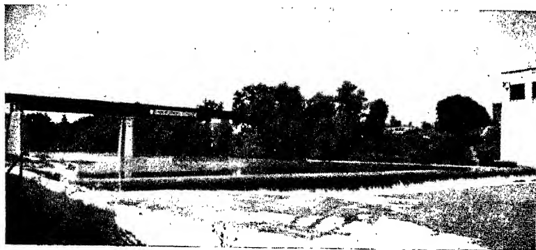
Fig. 9.—Dam at New Braunfels, Texas, built in 1922 with Limestone Coarse Aggregate. Continuously under Water with no signs of Deterioration.
